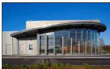
Usine eau potable
